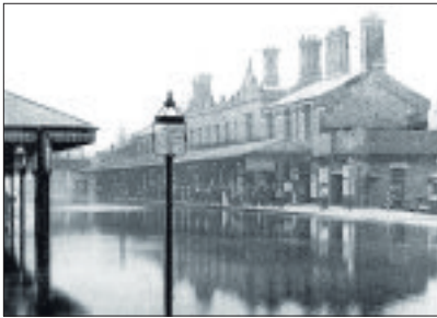
Walsall Station flooded by old South Staffs rail building
